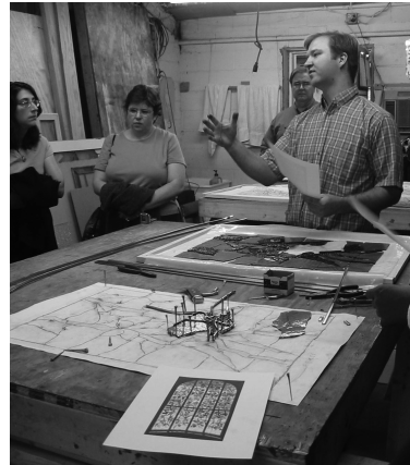
Jeff Loose, owner of Studio Glass, shows Trust staff how the stained glass window is being restored.
